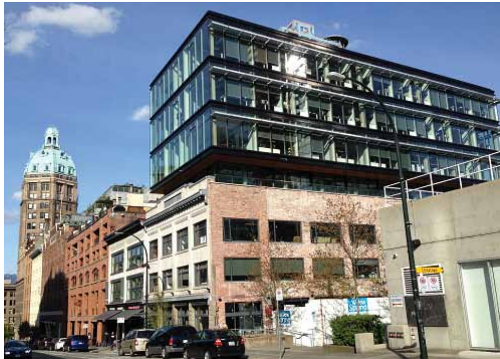
The new four-storey contemporary addition brings the 1909 heritage building into the 21 st century. Photo courtesy of Glen Stokes, Bruce Carscadden Architects Ltd.
